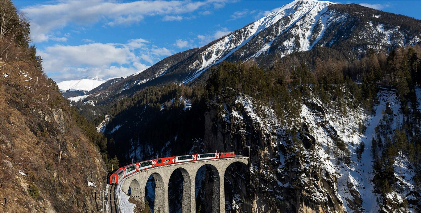
RhB Ge 4-4 II 614 Glacier Express on Landwasser Viaduct · Kabelleger / David Gubler · CC BY-SA 4.0 · cropped
